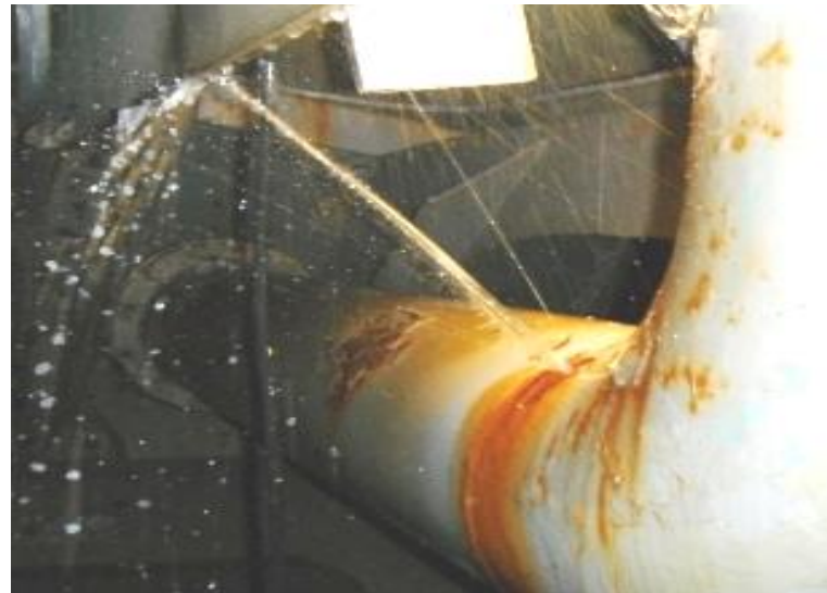
Ballast pipe – failure of internal coating
